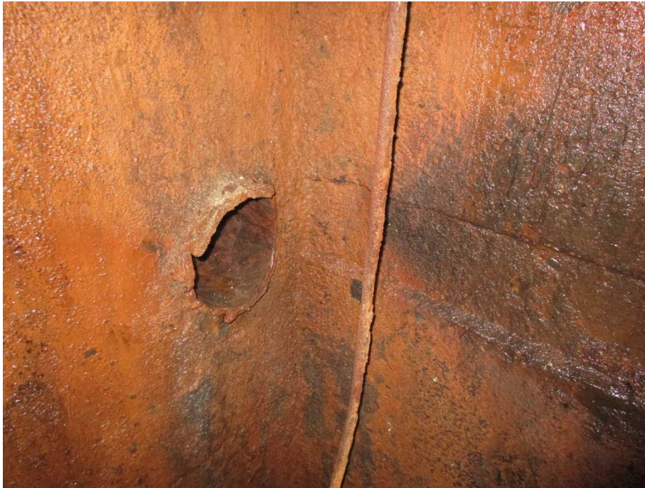
Photo 7 – Existing 8” pipe removed within interior of tower
